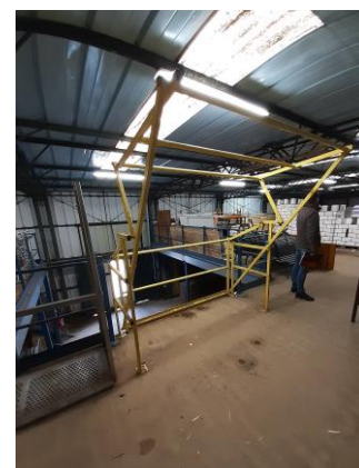
Mezzanine Services Techniques
