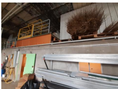
Mezzanine garage Services Techniques
